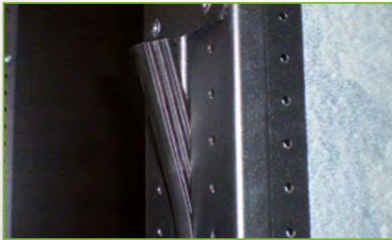
The inter-rack gasket ensures that your aisle is perfectly sealed.
